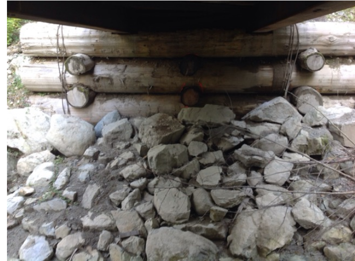
Right Bank Abutment when facing downstream
