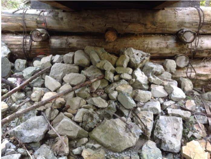
Left Bank Abutment when facing downstream
